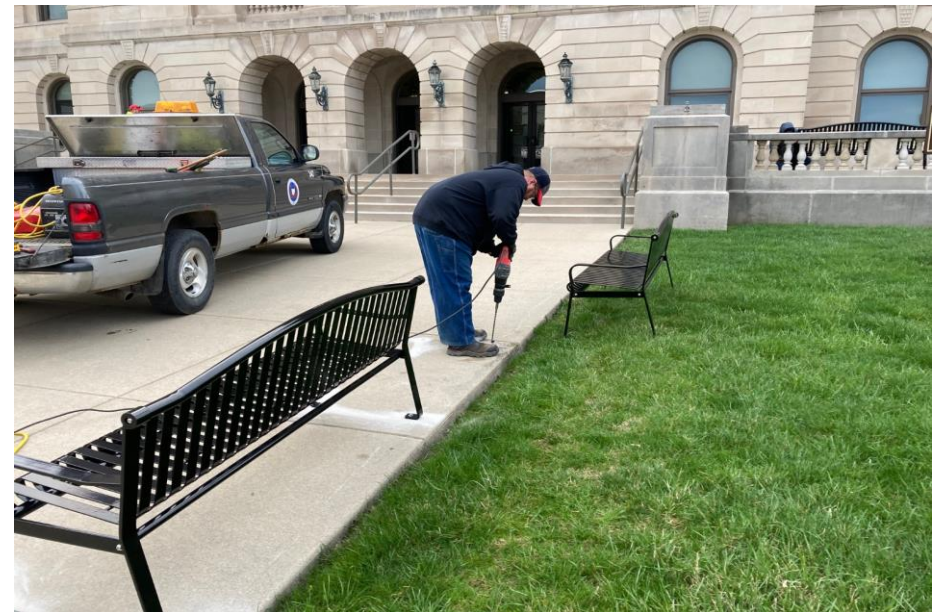
Crew installs Age Friendly benches on the Clinton County Courthouse steps
