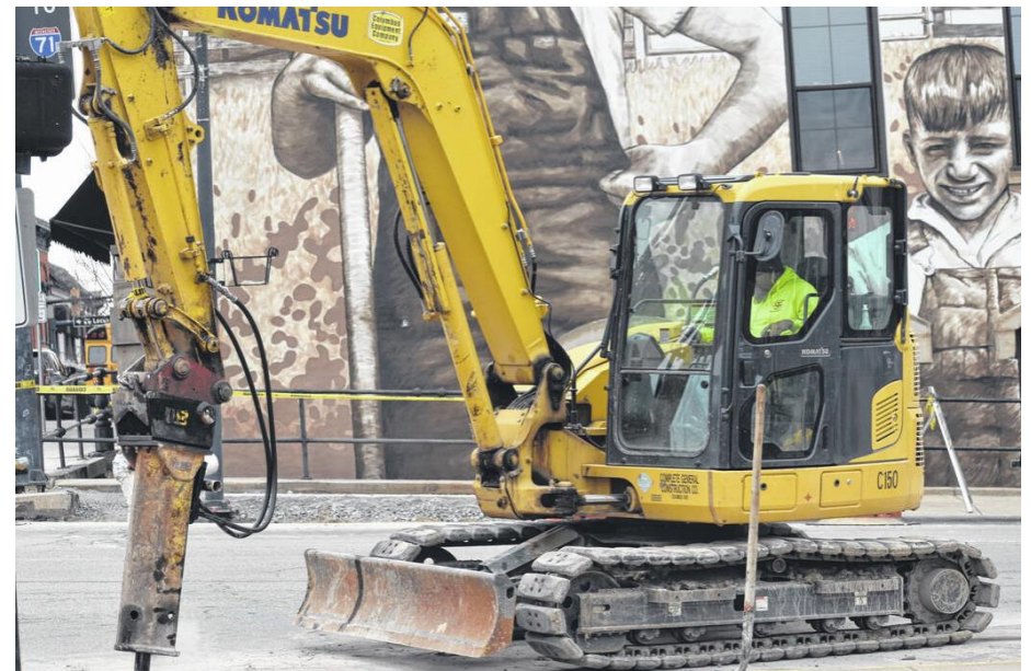
Crew installs bump outs in Clinton County, OH
