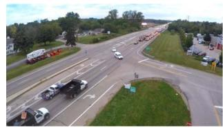
Factory and Orchard intersections into a Superstreet design: right turn only intersections from the side streets onto US 35 and the addition of signal controlled "U" turns through the median to accommodate the other directional movements.
