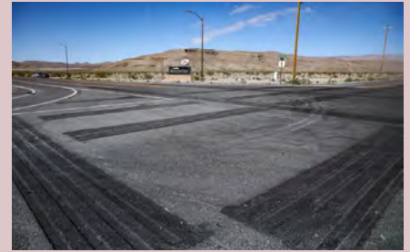
Transverse rumble strips placed before intersections help improve pedestrian safety in high speed areas.
