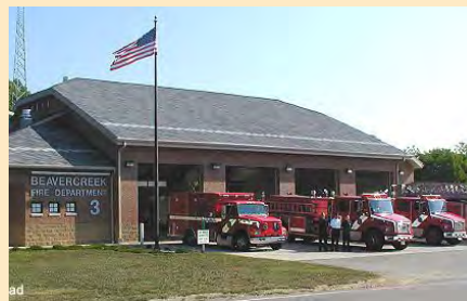
Leveraging existing community assets like churches or fire stations creates spaces for activity.
