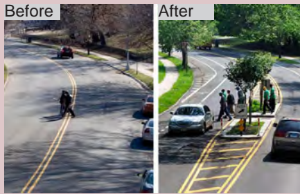
Introducing islands or medians improves the pedestrian environment for users of all ages.
