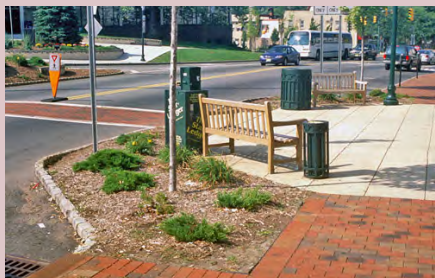
Bulb outs and other traffic calming measures improve safety for pedestrians.
